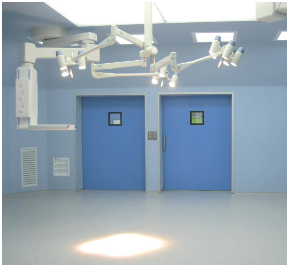
* Pressure Relief Damper in Modern Operation Theatre
